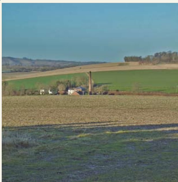
Crofton Pumping Station from the Roman Road. Photo by M Noyce.
