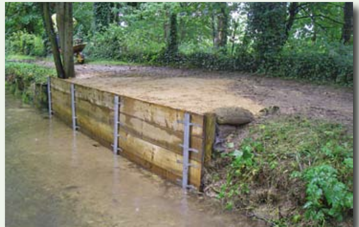
Bank erosion repairs, on the Thames Path at Ashton Keynes
